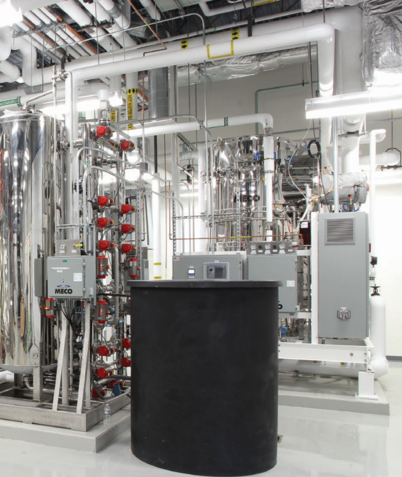
Pharmalucence WFI System and Clean Steam Generator
